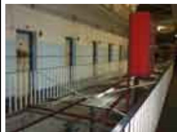
Level 2 East block
