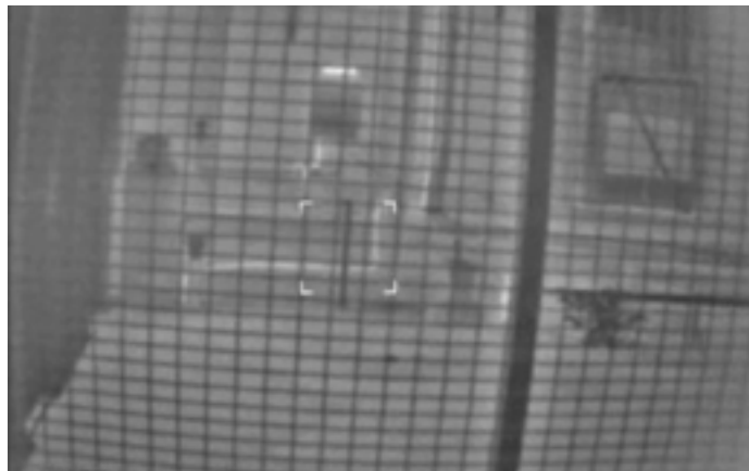
Thermal image from the courtyard area on level 1 near the shower block.
