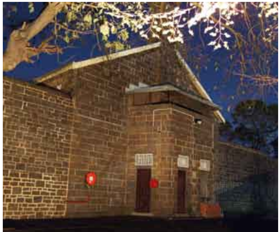
The end of the cell block from the exercise yard.
