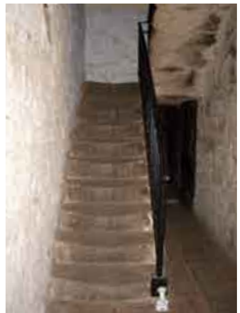
The stairs to the old kitchen where governor Fiddimont died in 1886.
