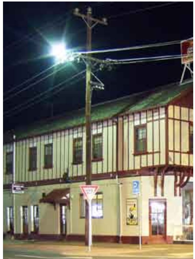
The hotels north-eastern side showing overhead mains power cable, street light and an underground power run, any of which could be contributing to the site's ambient EMF.
